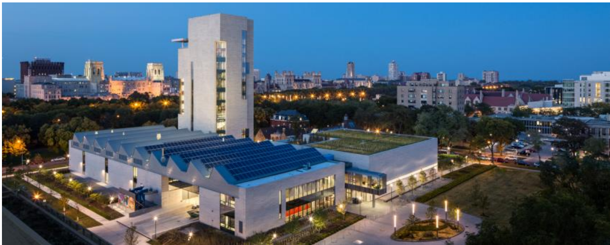
Figure 1: A façade of the Reva and David Logan Center for the Arts.
