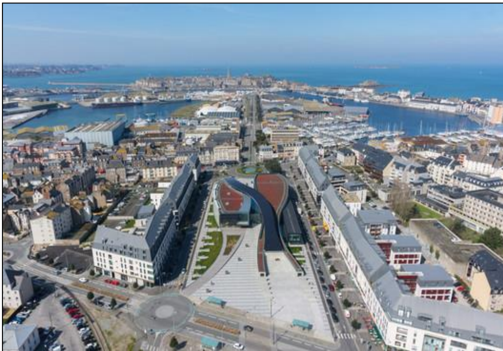
Figure 8. Eastern façade of St. Malo Cultural Hub
